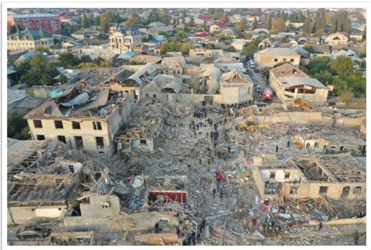
Photo 40 – 41 (next page): Destroyed residential area in Ganja (birdeye view)
